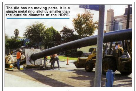
CML has served LADWP well in the past, but it is possible to get seepage through the material and that would exacerbate the existing external corrosion problem. A pressure-rated, cured-in-place technology is available, but in this case, it was prohibitively expensive. It would have cost almost as much as total replacement. After considering long-term serviceability, cost, and ease of application, a tight-fitting, high-density PE (HDPE) liner was specified for the rehabilitation projects.
